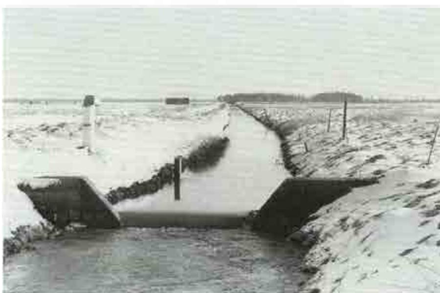
Fig. 4: The past of most Danish streams: Channelized, deepened, with weirs instead of riffles. This is now changed, in this stream too.
