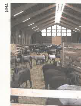
The recently built sheep shed at Hof Tütsberg is more translucent and pervious to air than old sheep sheds. At the same time, costs of fire insurance are lower than for the old sheds with their thatched roofs.
